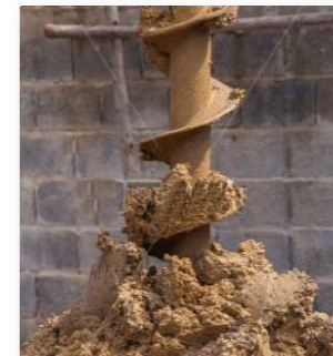
Foundation Drilling Auger
